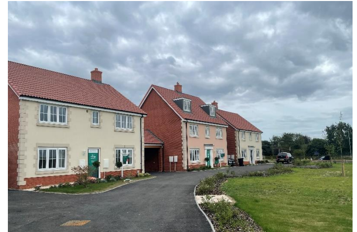
Dwellings at Site Entrance to Phase 1 – October 2023
