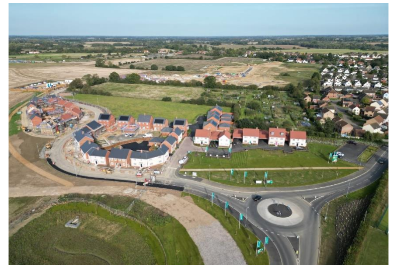
Drone images of build progress at Phase 1 – October 2023
